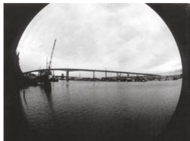
Images from the first 100 years: Exposing graft and improper contractor selection during construction of the West Seattle Bridge was a signature issue for the Municipal League in the 1970s. Photo: Steve Thornton
